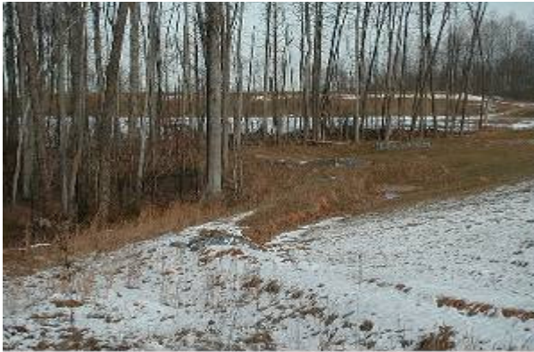
Diversion dikes can be used to contain storm water onsite
